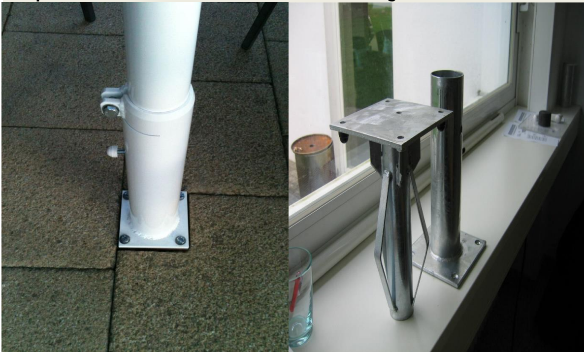
Tempest Upper Mast sleeve and galvanised steel ground anchor
